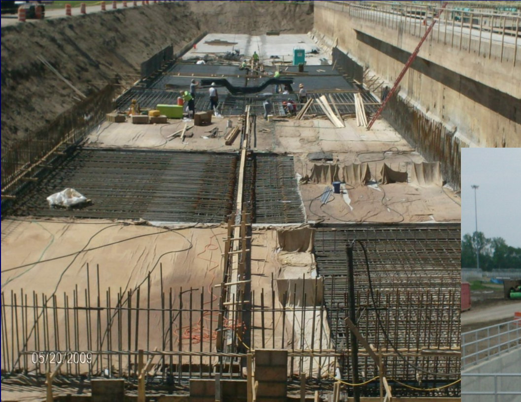
Tank A12 Bottom Slabs-on-Grade
