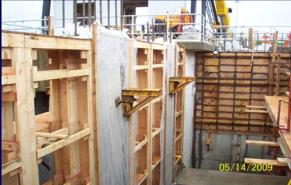
Effluent Pump Station Columns – May 2009
