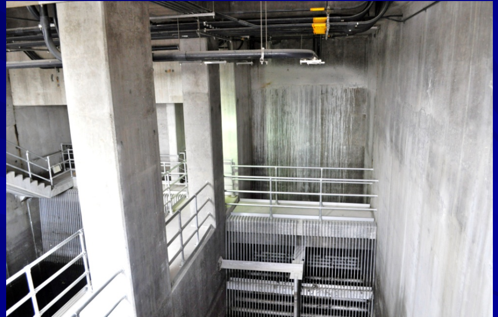
Effluent Pump Station Columns – May 2010
